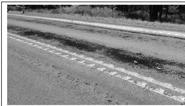
In Australia a big problem is melting asphalt as shown in the picture on the left. This is caused by melting bitumen from beneath the road's surface forced onto the surface by the pressure of vehicles, especially heavy vehicles, using the road. The road then presents with strips of slippery bitumen,
